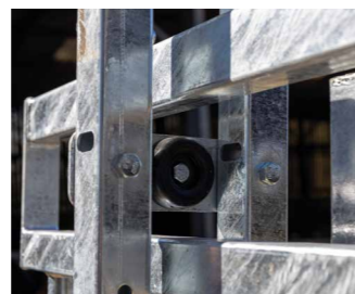
NOISE REDUCING RUBBER BUFFER
