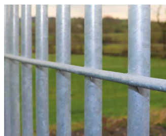
WELDED CROSS BAR FOR STRENGTH
